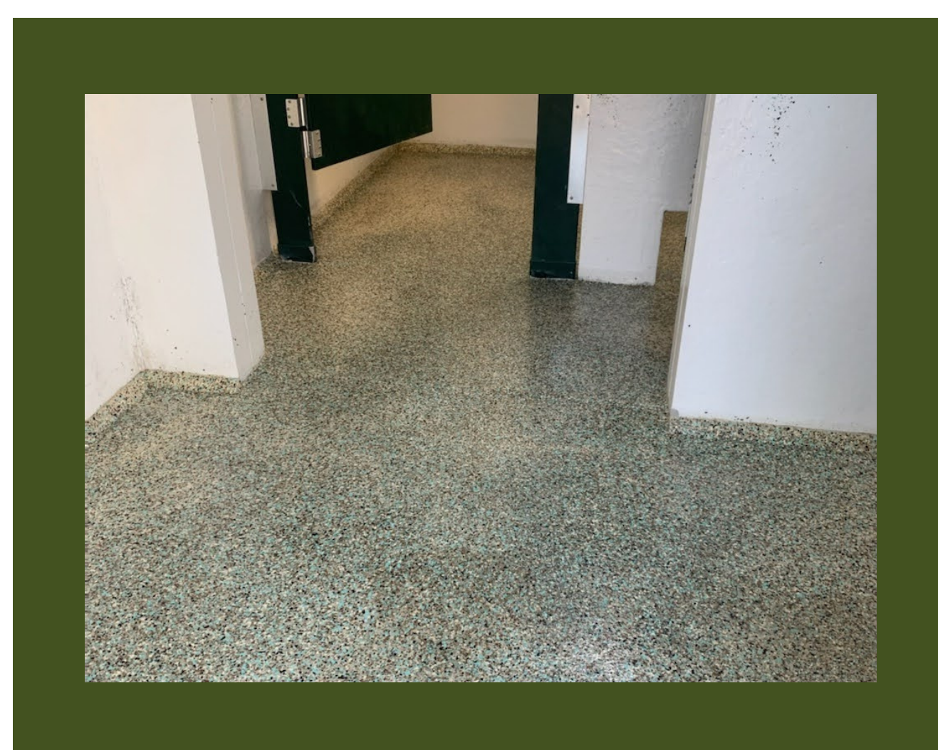
NEW EPOXY FLOORS AT PARK RESTROOM FACILITIES
